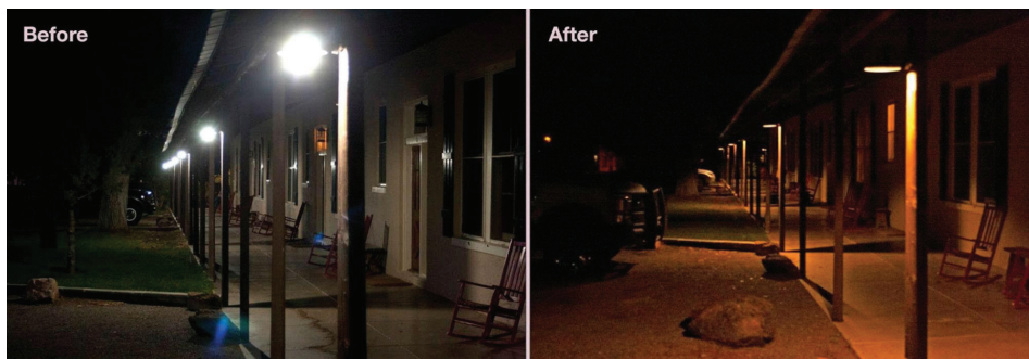
Photo 1. Before and after results for porch lights replaced with fully shielded fixtures.
